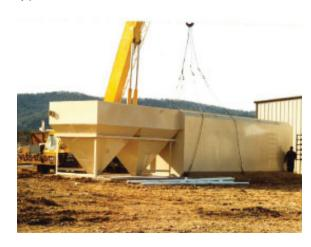
After setting the plant in position, check to be sure that it is level and in correct position.
