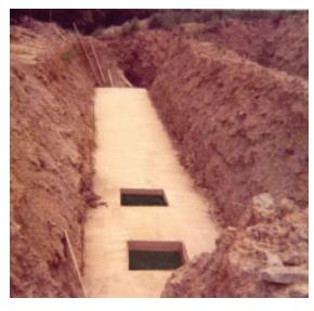
Notice the open areas in the foundation slab to accommodate the hopper cones.
