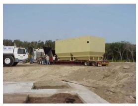
position the trailer, if possible, so that the hopper end of the tank will be placed at the discharge end of the pad. This will eliminate having to reposition the tanks later.
