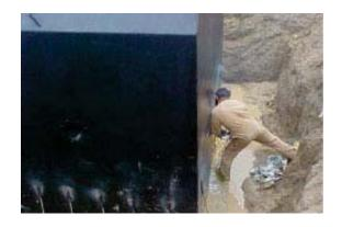
Reinforcing bars embedded into the concrete foundation pad are welded to the side of the tank walls to secure the plant and in some cases help prevent floatation.
